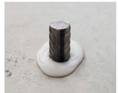
Figure 4-3: Freshly set rebar with HIT-FP 700 R
