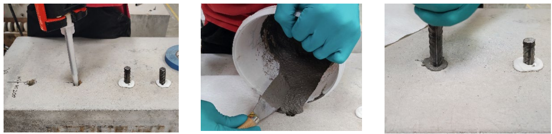
Figure 4-4: Installation of HIT-FP 700 R and generic grouts.
